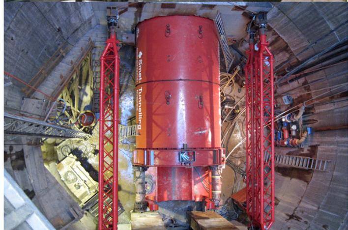
The pipes all have a steel core connected by welding after the pipe jacking is finished in order to drain a watertight tunnel. At such depths a standard concrete wall of 24 cm is not sufficient enough to guarantee watertightness because of the water pressure.
