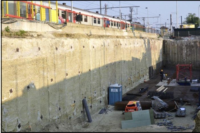
**Ground nailing consists of placing a number of nail-like reinforcing elements in the ground to absorb stresses in the ground. Ground nailing creates a reinforced ground body. A layer of shotcrete approximately 10 cm thick is usually sufficient cladding for a ground body reinforced in this way.**
