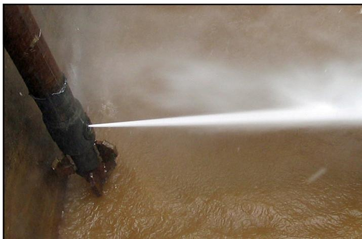
**Very high pressure (VHP) grouting, also called jet grouting, involves the in situ mixing of soil with water and cement to form grout columns that can be used for foundations, general soil stabilisation, earth retaining or anchoring. Grout columns can be formed underneath existing walls and/or foundations by using relatively small-diameter drilling rods.**
