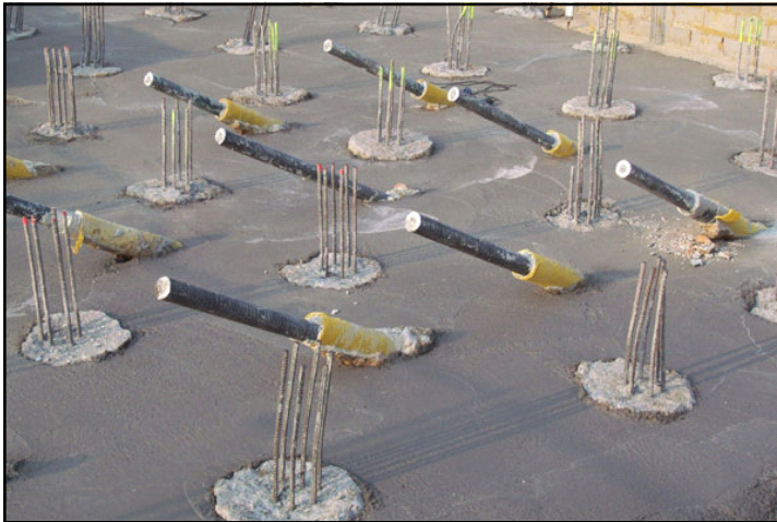
Micro piles are small-diameter piles with relatively high load bearing capacity.
