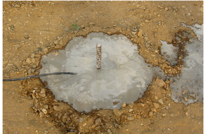
Micro piles are small-diameter piles with relatively high load bearing capacity.
