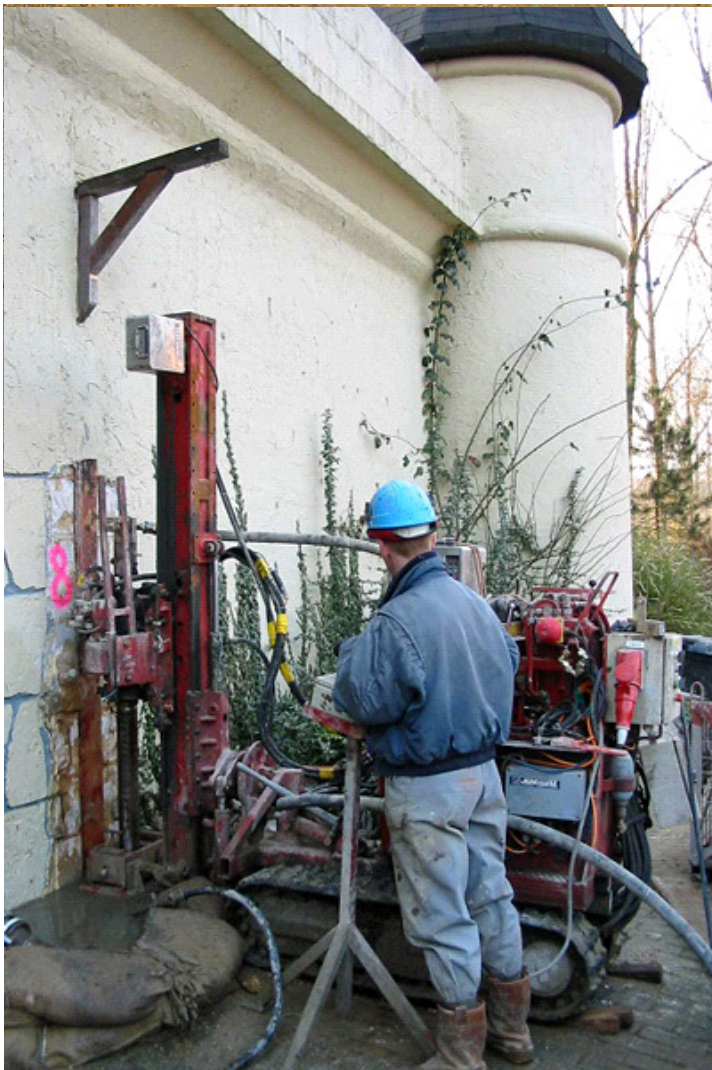
Micro piles are small-diameter piles with relatively high load bearing capacity.
