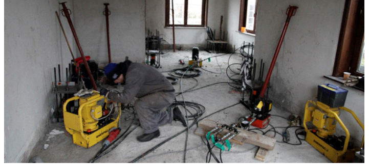
Injections can be used to fill cavities and pores in the sub-soil.
