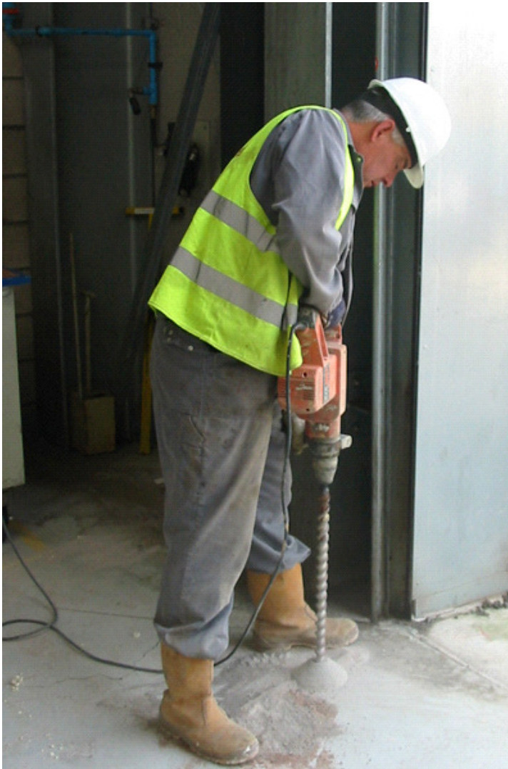
Injections can be used to fill cavities and pores in the sub-soil.
