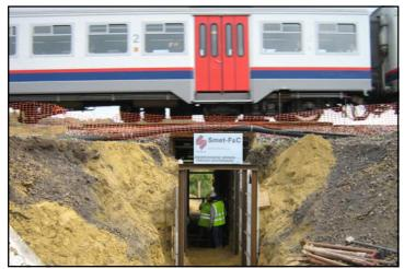
"Timbering" literally means covering with wood or stone. This technique has been used for ages in mining, where trenches are excavated in stages and the ground is supported by concrete panels that are held in place and aligned to each other by steel shores.
