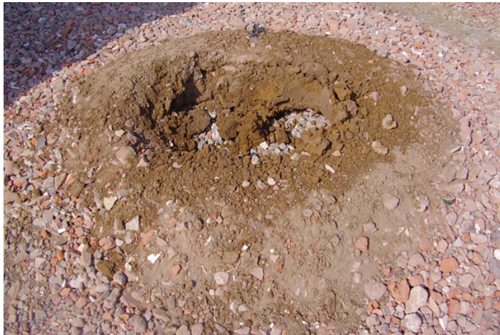
Gravel cores forming the foundation for floor slabs.
