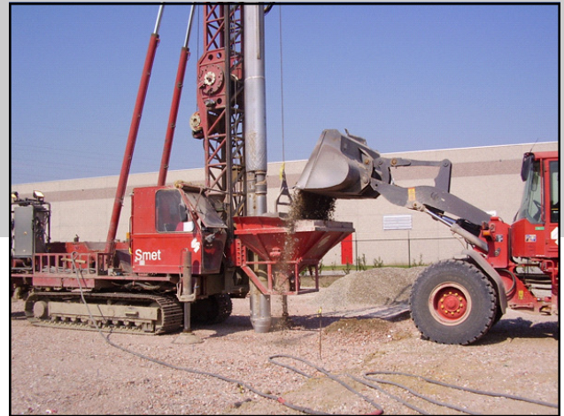
Gravel cores forming the foundation for floor slabs.
